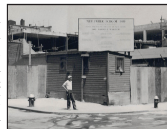
Construction of the Nathan Straus School, P.S. 140 1959
